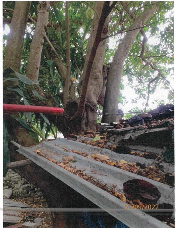
T06 - Decay On Branch(F)
