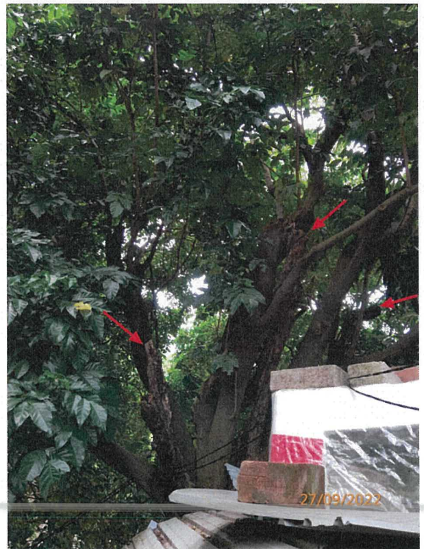
T04 - Decay Brnaches(F)
