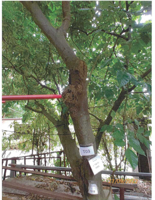
T03 - Decay On Branch(F)
